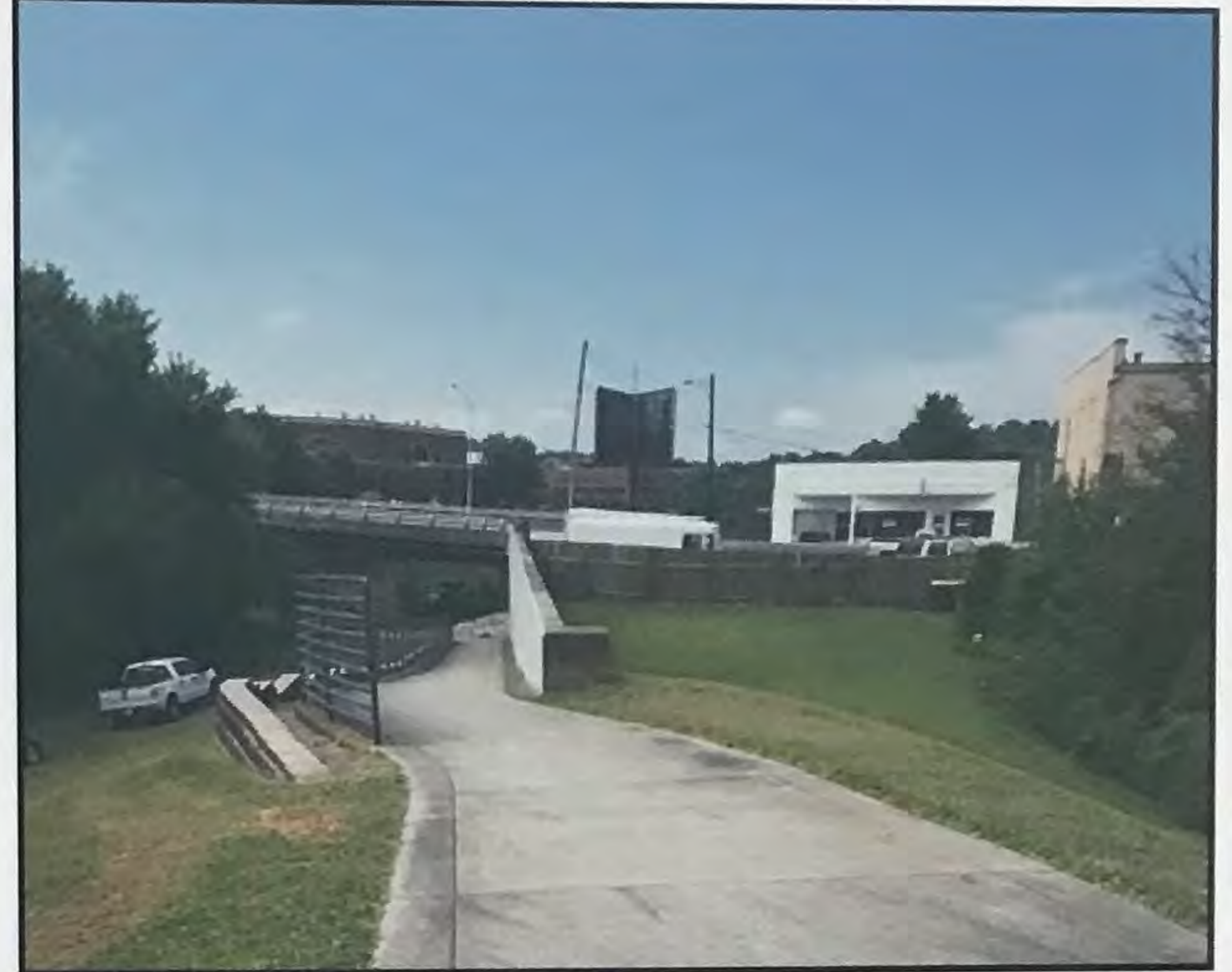
Floodwall tie-in at Rome, GA Levee.
