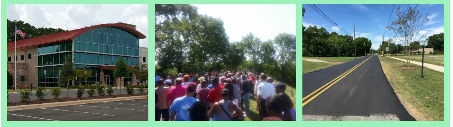
(left to right) The Western Health Clinic, the High Ore Trail, and new paving along Martin Luther King, Jr. Drive to compliment the new sidewalk.
